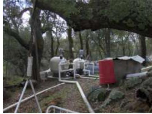
Marilee's 2 bubble bead system, pre-filter, and UV (under red tub) was installed by Mamason Koi of Grass Valley.
