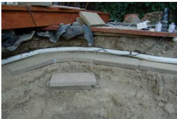
One of the earliest thoughts that was driven in to us by club members was the role played by friction and loss of water flow due to elbows and undersized pipe. Most of our pressure lines are 2" or larger. One of the tricks we learned was to heat up PVC pipe with an inexpensive heat gun from Harbor Freight (less than \$15) and carefully form it to the desired shape. This took a little extra time but eliminates or minimizes the use of elbows and friction.
