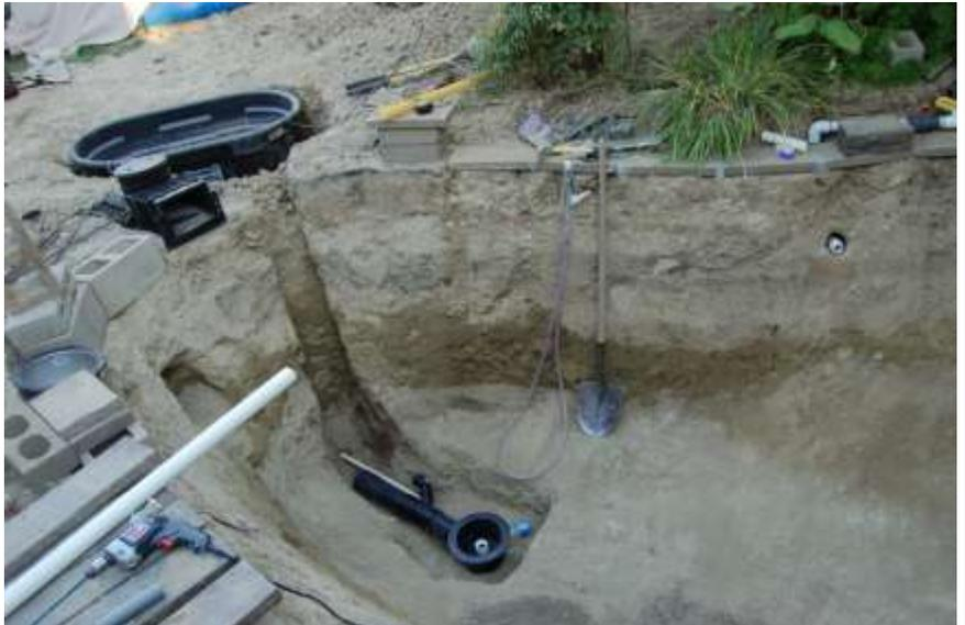
The bottom and sides of the pond were shaped carefully so any debris would naturally flow to the drain.
